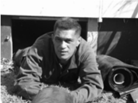
Horace Pehi emerges from under a newly insulated home.
