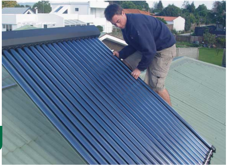
| Installing a solar water heating system.
